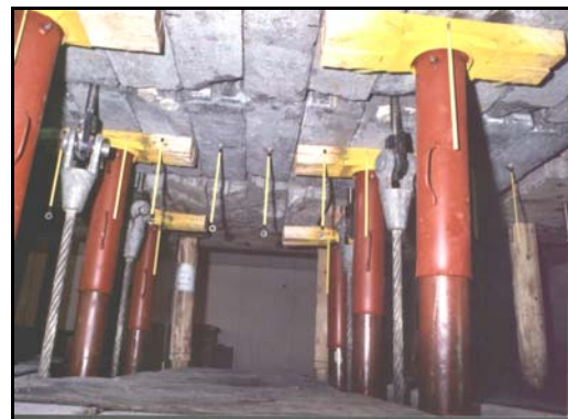
Figure 2: The support system before the first drop test from a height of 1.2 metres.
