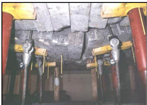
Figure 10: The hangingwall beam condition after the second drop, showing the central beam deflection.
