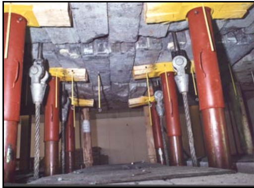
Figure 4: The conditions of the props and hangingwall beam after the first drop test.
