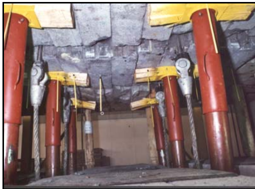
Figure 5: The condition of the hangingwall beam and props were still good after the second drop.
